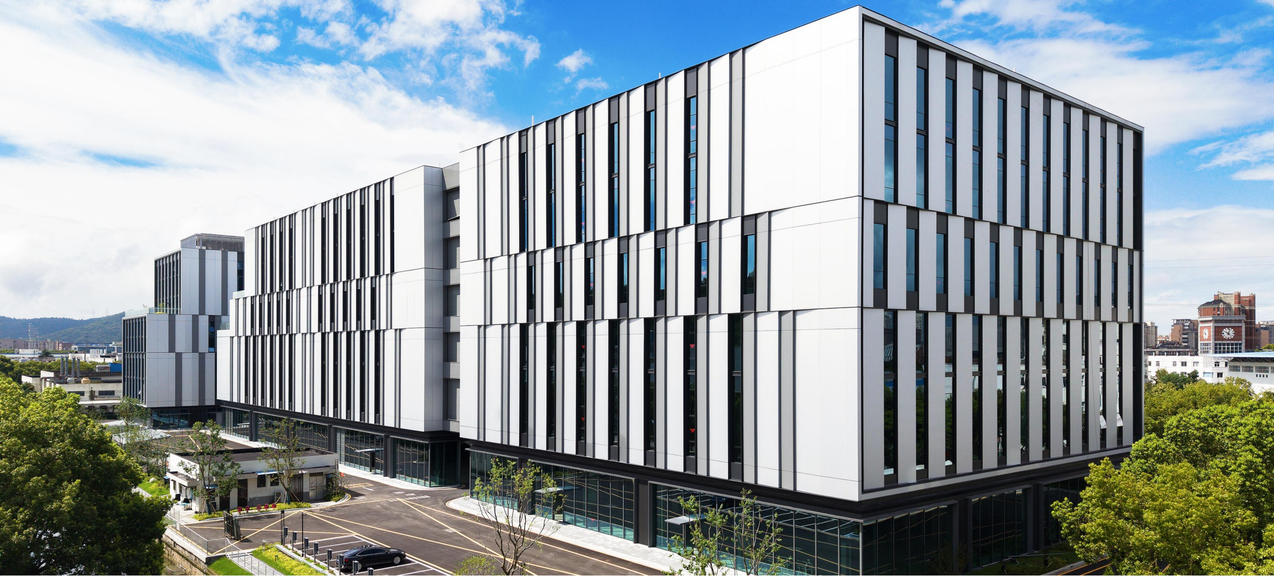
■ Suzhou Hengshan Intelligent Manufacturing Factory 苏州横山智造工厂
